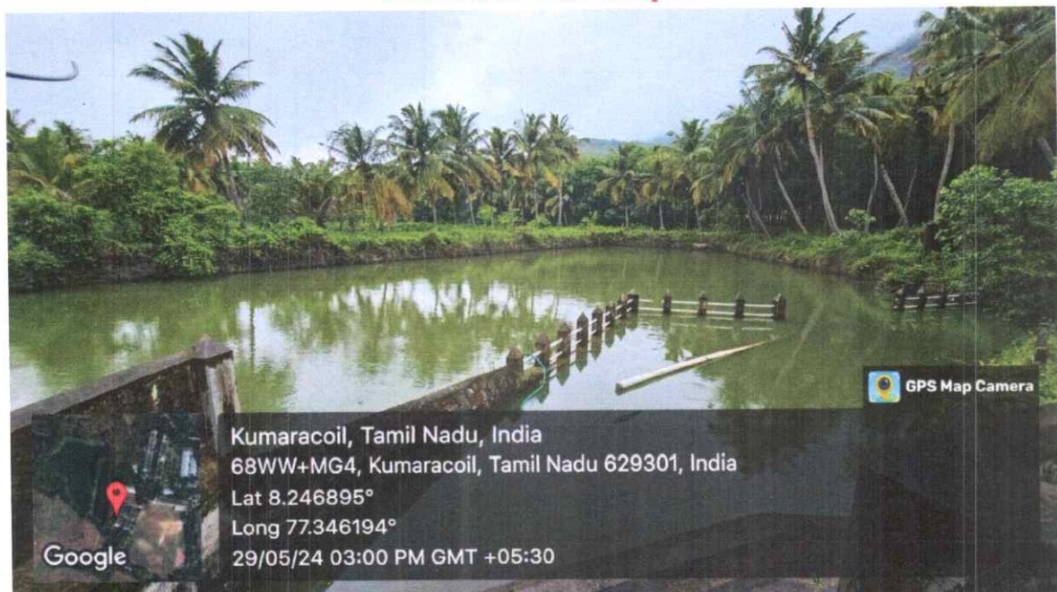
Water Bund in the Campus
