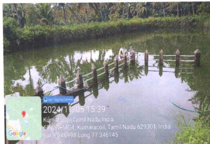
Water Storage bund
