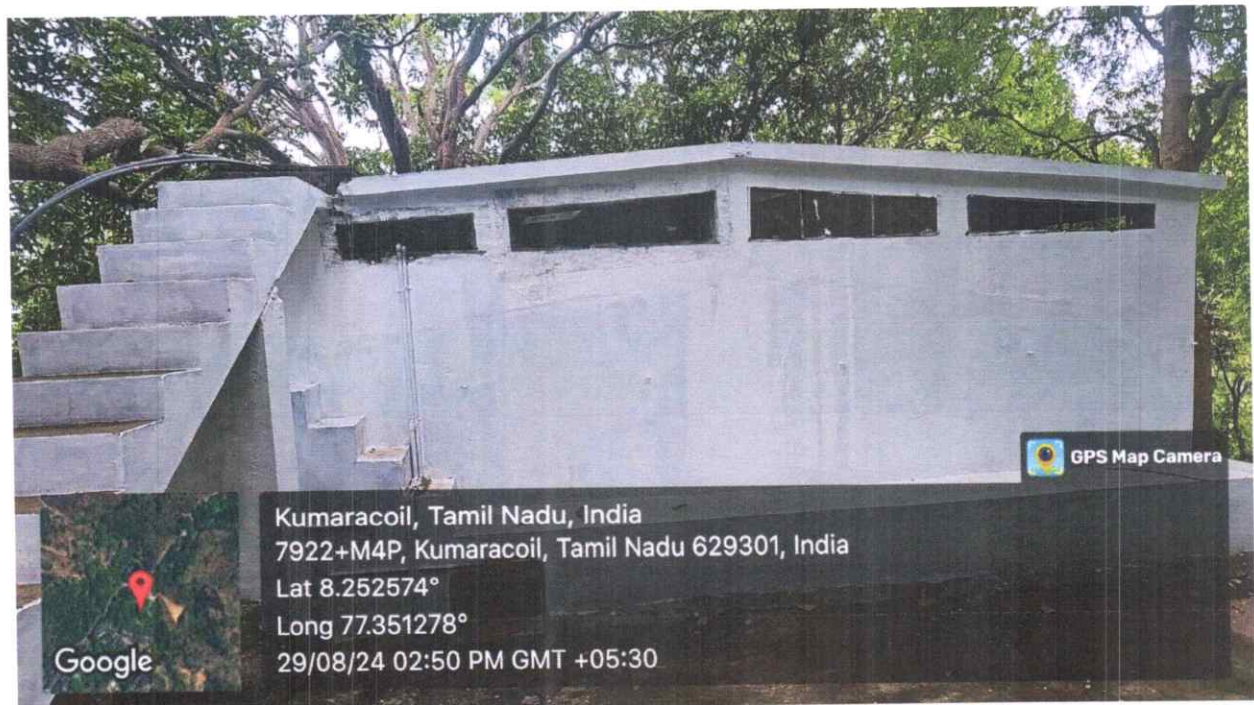
Water Tank with a capacity of 1,30,000 litres
