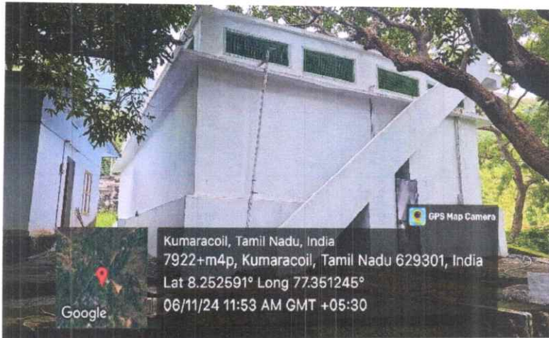
Water Tank with a capacity of 4,30,000 litres
