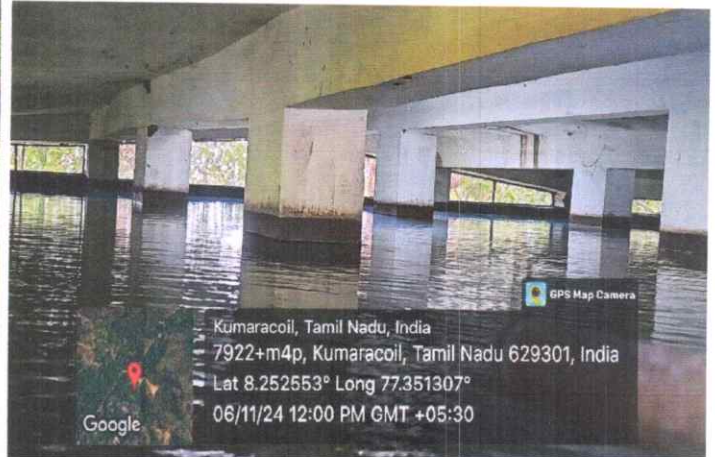
Water Stored inside the Tank with a capacity of 4,30,000 litres
